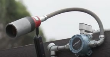
Hydrogen Sensor - if detection hits a certain level, triggers alarms or shutdown of equipment
